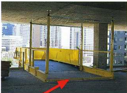
TIE BAR IN POSITION FOR LIFTING AND TRANSPORT
